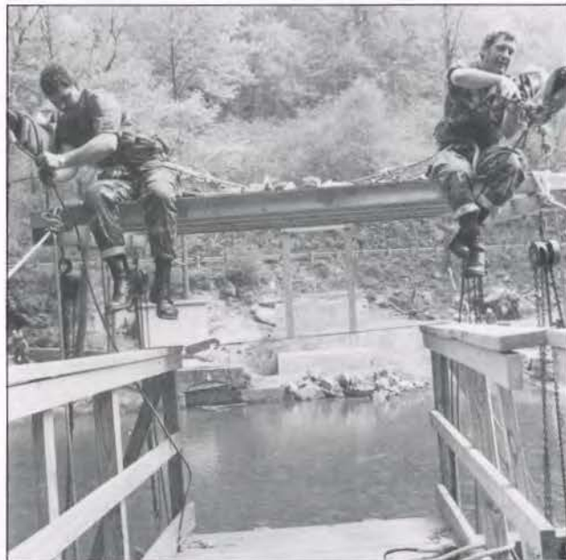
Spec. Mark Lucas, left and Sgt. Michael Wood of the Maryland Army National Guard's Company B, 121st Engineer Battalion tighten the vertical support cables holding one of the bridge sections in place in preparation for the Maryland International Canoe/Kayak Classic at the Savage River in Garrett County. (Photo by 1st Lt. John Goheen)
