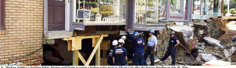
Workers stabilize a building before digging could begin to repair a broken water main in Ellicott City after the historic flooding on July 30, 2016.
