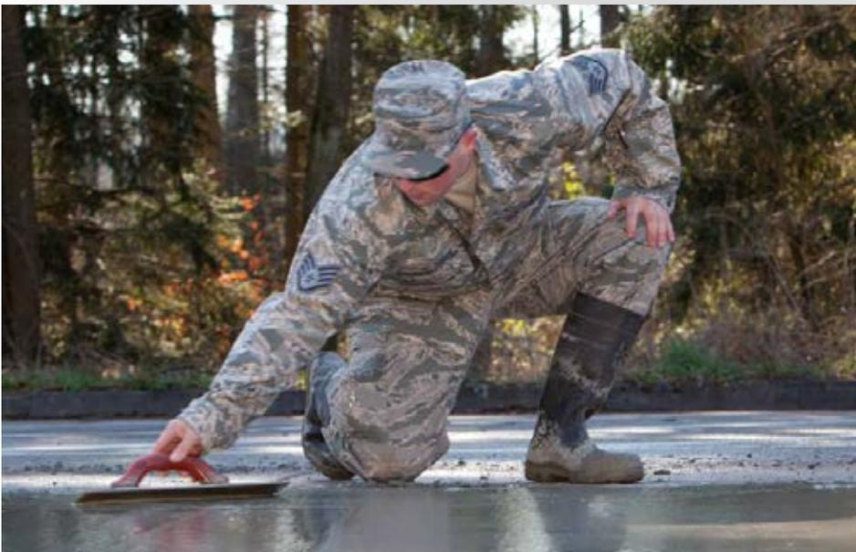
Air Force Staff Sgt. Steven Unglesbee, 175th CES, uses a bull float, a cement-finishing tool, to even out the surface of a concrete pad during the construction project portion of the Silver Flag exercise, March 24, 2014.
