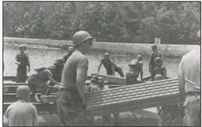
Members of the 121st Engineer Battalion assemble a pontoon bridge during annual training at Fort A.P. Hill, Va. (Photo by Maj. Howard S. Freedlander)
