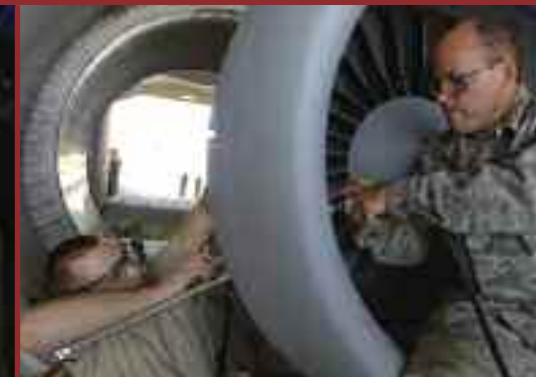
Staff Sgt. Jonathan Pollack, 438th Air Expeditionary Group structural maintenance technician, (left) and Master Sgt. Anthony Bahur, structural maintenance supervisor, perform a structural repair on an A-10C Thunderbolt II's engine inlet. (U.S. Air Force photo/Tech. Sgt. D. Clare)
