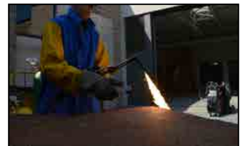
Senior Airman Andrew Bracken, structural journeyman assigned to the 175th Civil Engineer Squadron, Warfield Air National Guard Base, Middle River, Md., lights an acetylene torch in preparation for a demonstration in raw cutting steel for fabrication purposes, Sept. 6, 2014.
