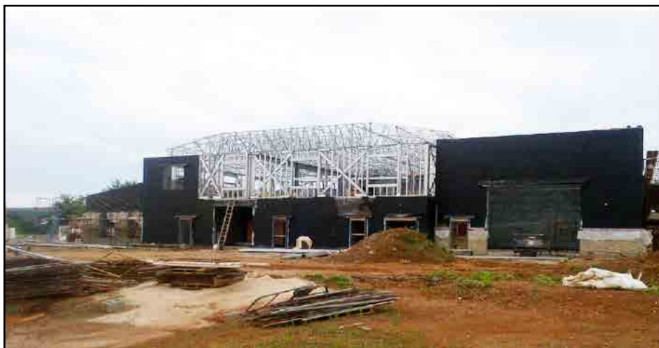
The renovation of the Westminster Readiness Center is 100 percent federally funded at a cost of $7.9 million and is scheduled for completion in early in 2015.
