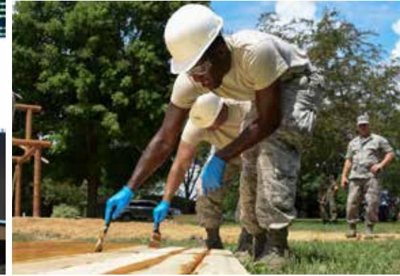
▲ 175th Wing Civil Engineer Squadron collaborate with service members of the Armed Forces of Bosnia and Herzegovina during a demolition exercise PATRIOT North 17, on July 18, 2017, at Volk Field, Wisconsin.
