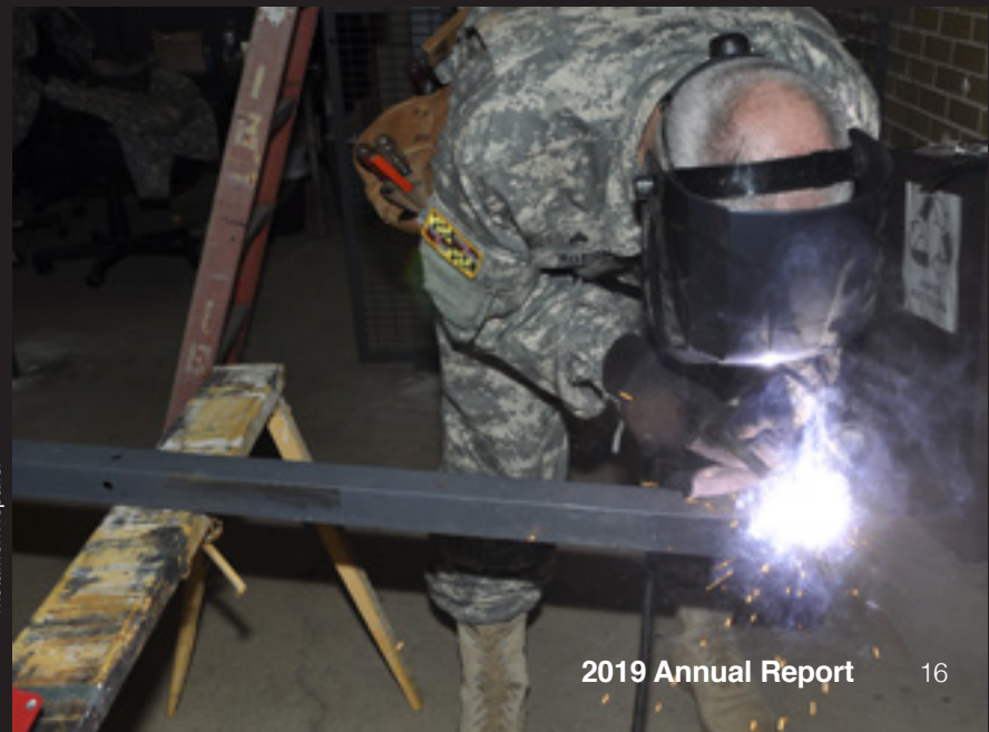
A member of the MDDF's 121st Engineer Regiment performed metalwork repairs.
